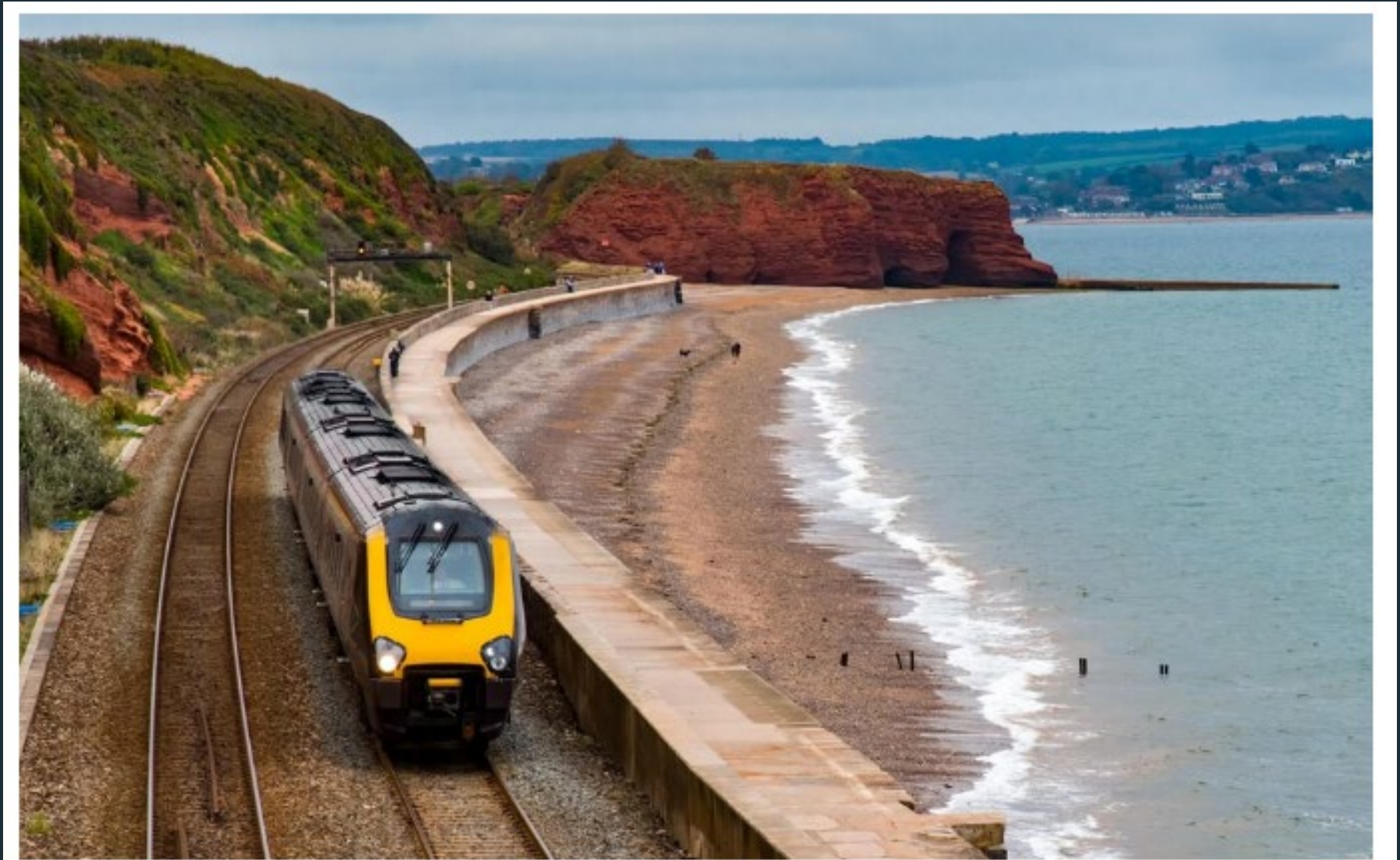
There is 650km of railway line at risk from coastal erosion according to the Climate Change Committee Credit: Paul Martin / Alamy Stock Photo
