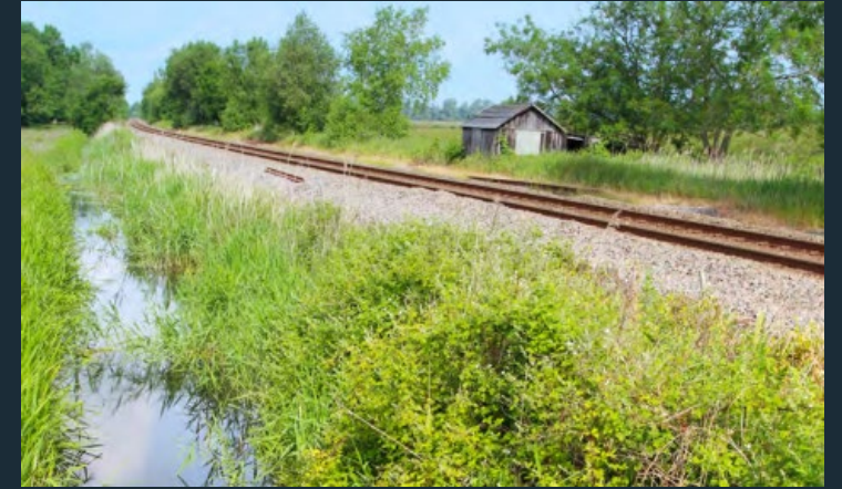
Drainage channel and wetland adjacent to the rail corridor, Anglia Route, Eastern Region.
